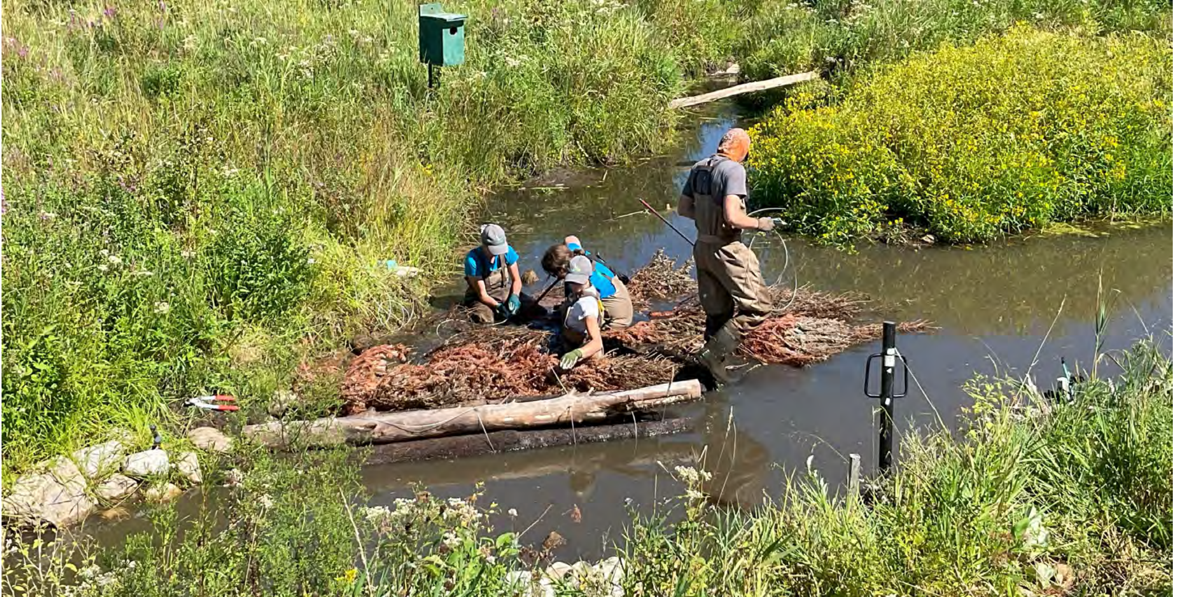
Recycled Christmas trees made excellent sediment mats and were biodegradable.
