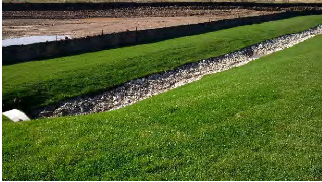
Temporary channel lined with rocks
