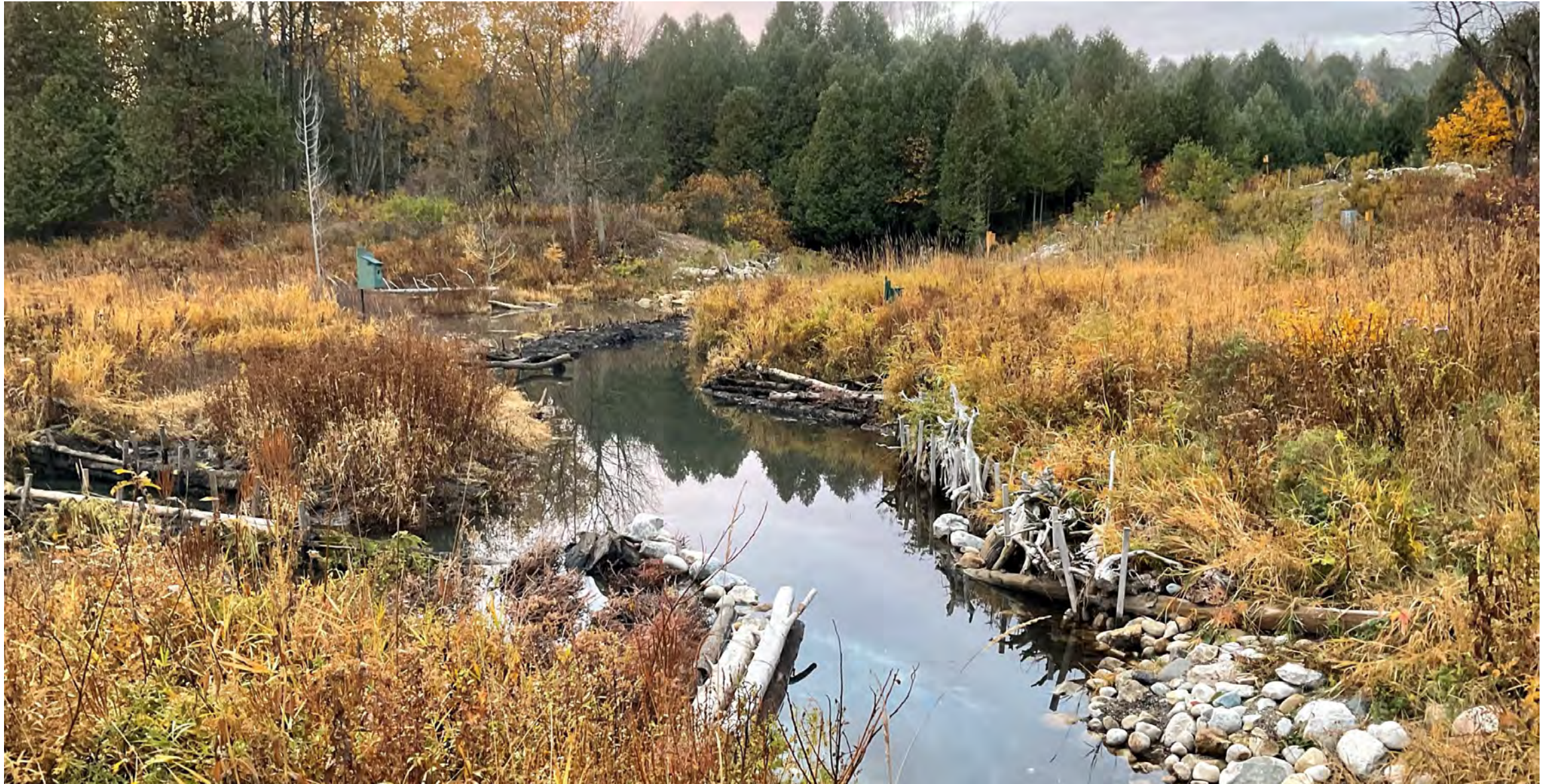
Conservation Halton staff installed sediment mats and log structures to shape the creek.
