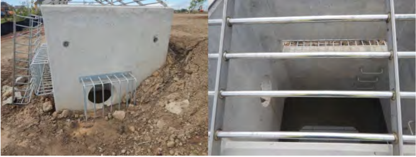
FIGURE 3-2: EXAMPLE OF DESIRED OUTLET CONTROL COMPONENTS
