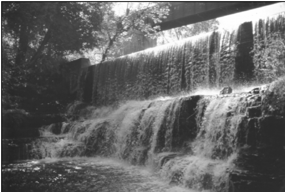
Progreton Dam, Bronte Creek
