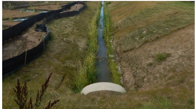
Temporary channel bed lined with vegetation
