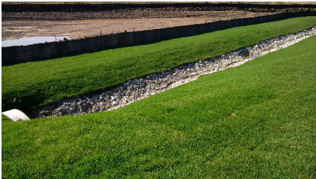
Temporary channel lined with rocks
