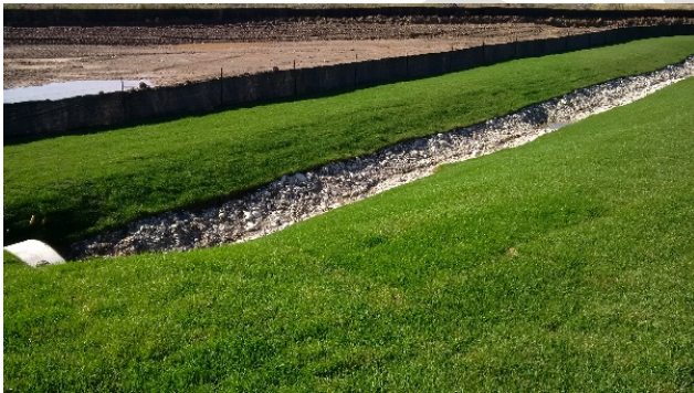
Temporary channel lined with rocks
