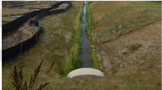
Temporary channel bed lined with vegetation
