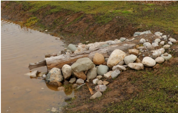
Example of instream habitat built into the creek bank
