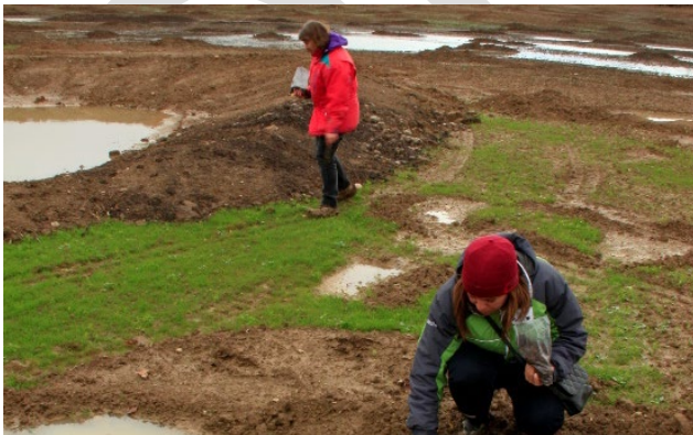
Seeding during construction of pit-and-mound features
