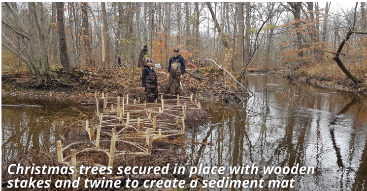
The online pond has been separated from the creek with the sediment mat
