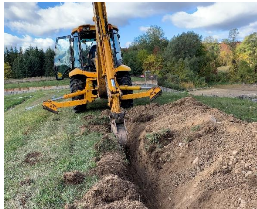
CONSTRUCTION OF SUB-DRAINAGE SYSTEM TO REDUCE HYDROSTATIC PRESSURE AT SCOTCH BLOCK DAM
